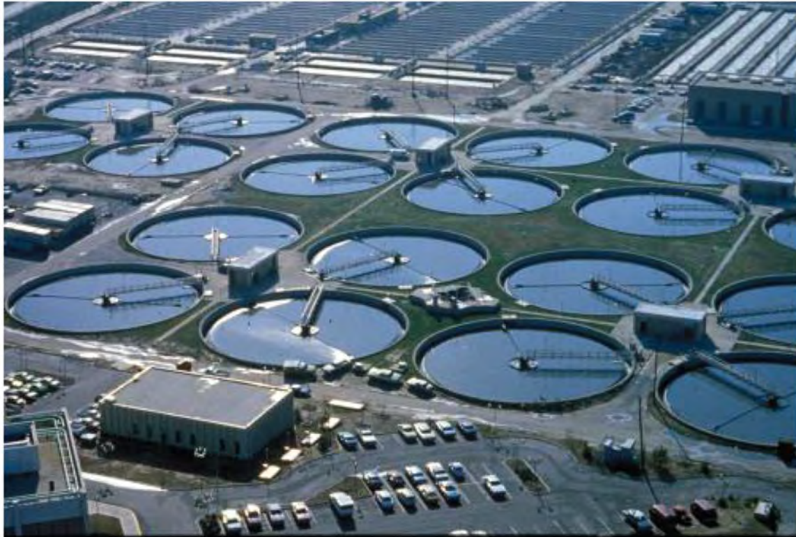
Figure 25.1 Sewage Treatment Plant (credit: "eutrophication&hypoxia"/flickr.com)
